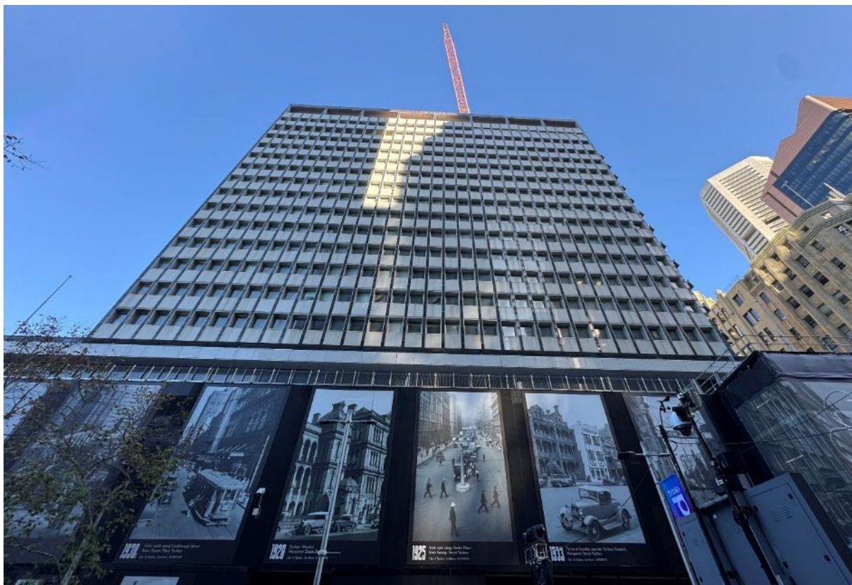
Figure 3: Site viewed from Martin Place
